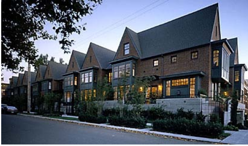
The Victoria Townhomes were designed to blend in with and play off of the historic architecture of the neighborhood, particularly that of the adjacent Victoria Condominiums.
